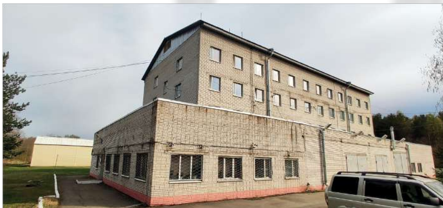
FIRE ALARM CENTER 131 Otradnoe village
